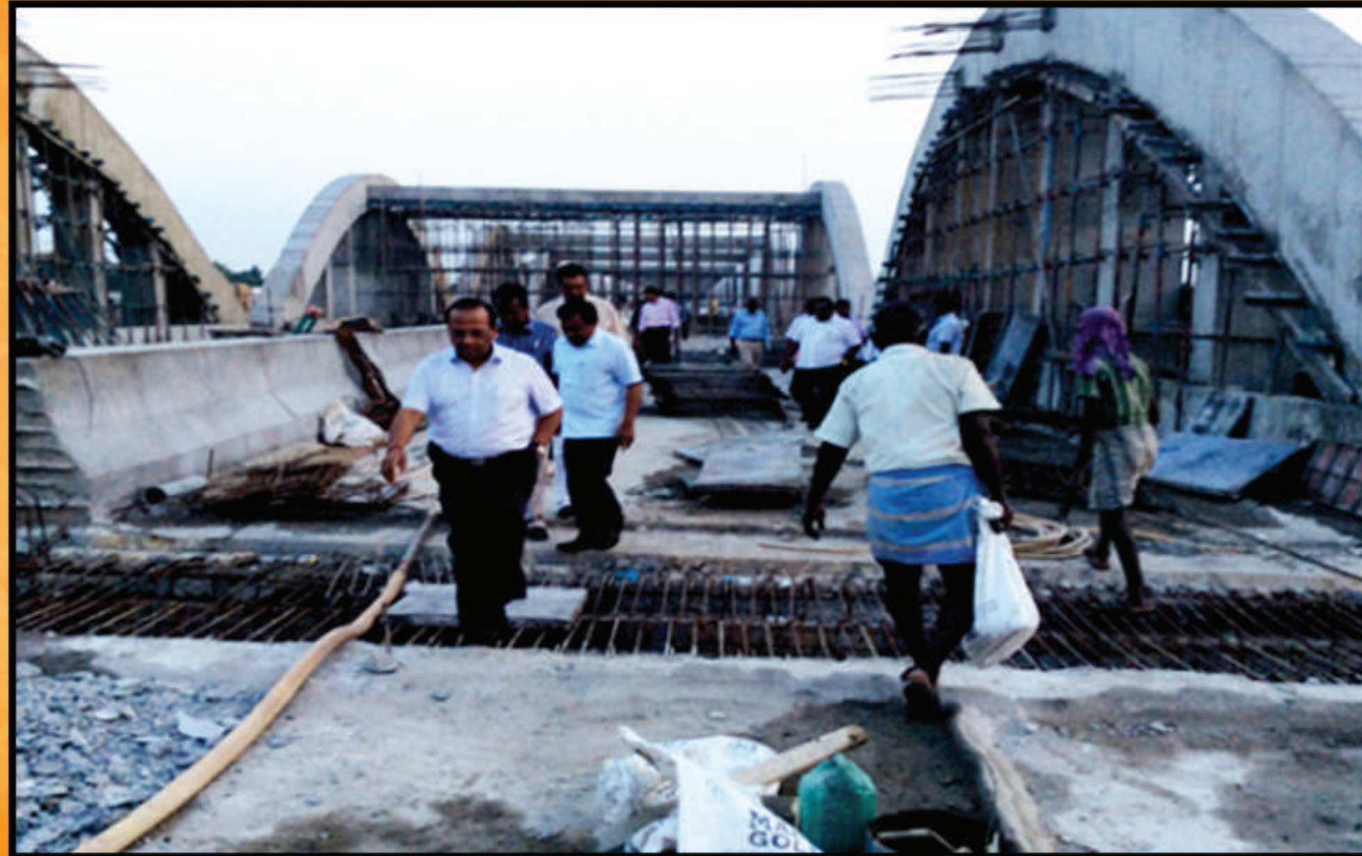
Inspection of the Chief Engineer K. JAYARAMAN, Kollidam Bridge, Trichy.
